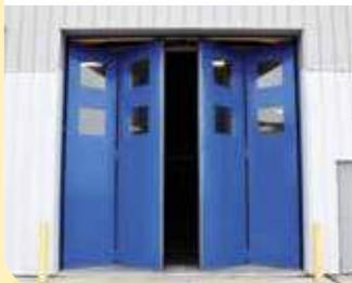
Four-fold doors open vertically rather than horizontally and are ideal for buildings housing emergency response vehicles, such as fire stations.
