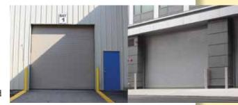
of Missile Level E as specified in ASTM E 1996-14a. Extreme 300 Series and Extreme 1024 High-Performance rolling doors are operational up to 10 PSF maximum wind load, and the Extreme 300 Series door remains static in up to 50 PSF design wind load. These results comply with TDI standards assuring the doors remain secure and can resist high pressure, intense weather situations. <a href="https://www.cornellcookson.com">www.cornellcookson.com</a>
