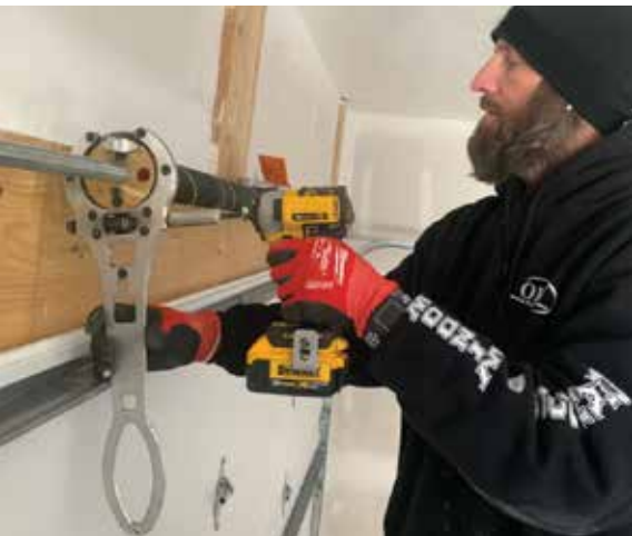
Implementing spring winding tools was an engineering change that helped the company reduce long term rotator cuff damage.
