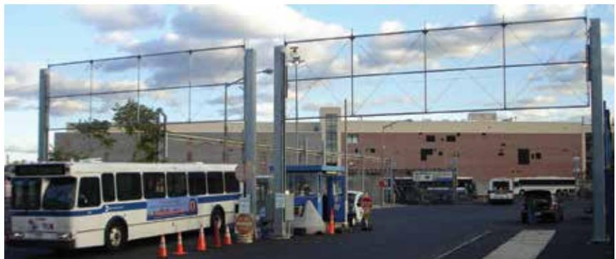
There are also several other added benefits as well. Vertical lift gates are quite fast compared to swing or slide gates with similar lane widths. A secondary barrier arm gate is a good idea for these situations to prevent trucks with high cargo loads from crossing the access point until the panel is fully open.
