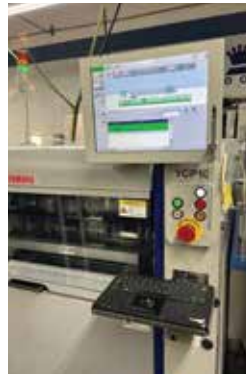
The computer control for the surface mount machine.
