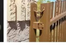
Adding a fall-over post and a cable or chain, to collar the top of the gate, can prevent the gate from falling over.
