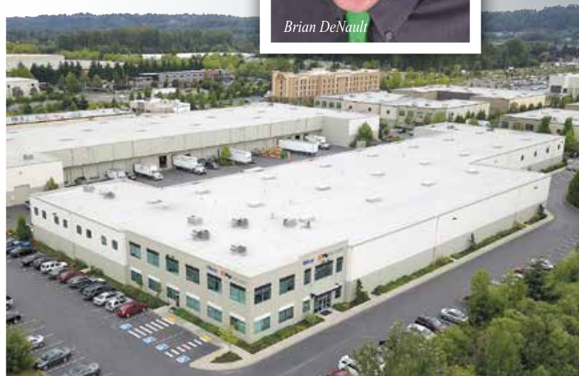
HySecurity's new headquarters, Kent, Wash., 2018.
