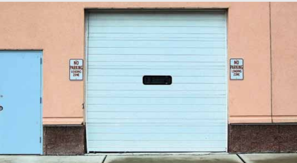
THE DOOR: The accident occurred at the left side of this door. The stepladder had been placed under the open door, in the doorway. (Photo by Dynamic Evidence of Fort Lee, N.J. Used with permission.)
