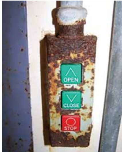
This NEMA 1 station was installed in a wash bay and used for three years. Always remember that water and electricity don't mix.
