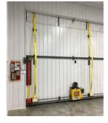
The new hydraulic-door wind pin locks the door to the building. Pushing the up/down control button opens or closes the door and sets the wind pin in place. *www.schweissdoors.com*
